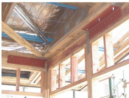
■ Typical connection to bracing wall.
