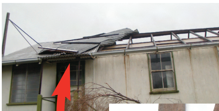
■ Inadequate batten to rafter fixing.
