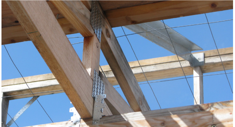
■ A kneebrace to a parapet.
