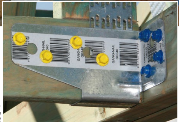
■ Photo 2 - Colour coded screws fixing a Girder Bracket
