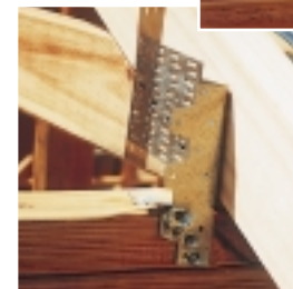
Too many nails, too much pressure, too little pressure, too close together, too close to the edge - we have it all here.
