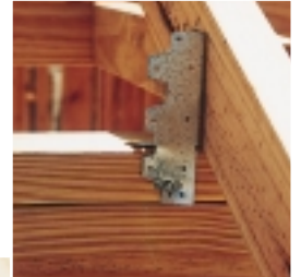
The two nails on top have missed the timber plate altogether.
