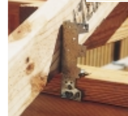
Attempts to nail through pre-punched holes only tear the holes and result in loose and weakened connections.
