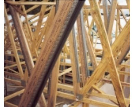
■ *Web stiffeners should be used in preference to web ties where the webs to be braced are not in alignment.*
