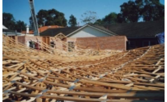
or "Speedbrace" as temporary brace, which works well as a tension brace but has no compressive capacity so is the opposite problem to the nogging system.
