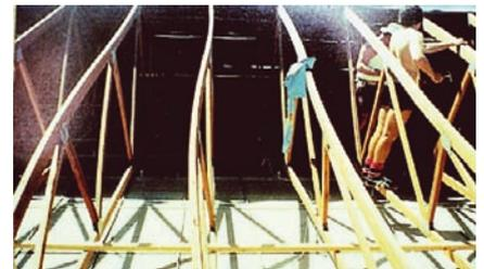
The correct installation and fixing of temporary bracing will help avoid these failures and provide a straighter and safer roof structure.
