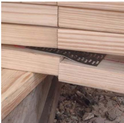
*Poor bundling and stacking of trusses causing nailplate failure.*
