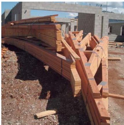
*Laying trusses on uneven ground causes distortion and unwanted stresses to build.*
