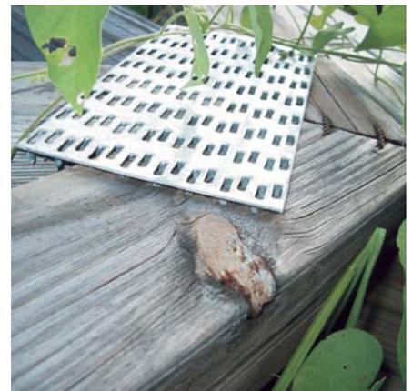
*Prolonged exposure to weather causing timber splitting and joint failure.*
