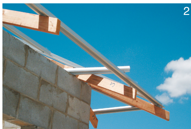
■ A worker risked injury to install these battens on a hip corner not supported by a structural fascia.
