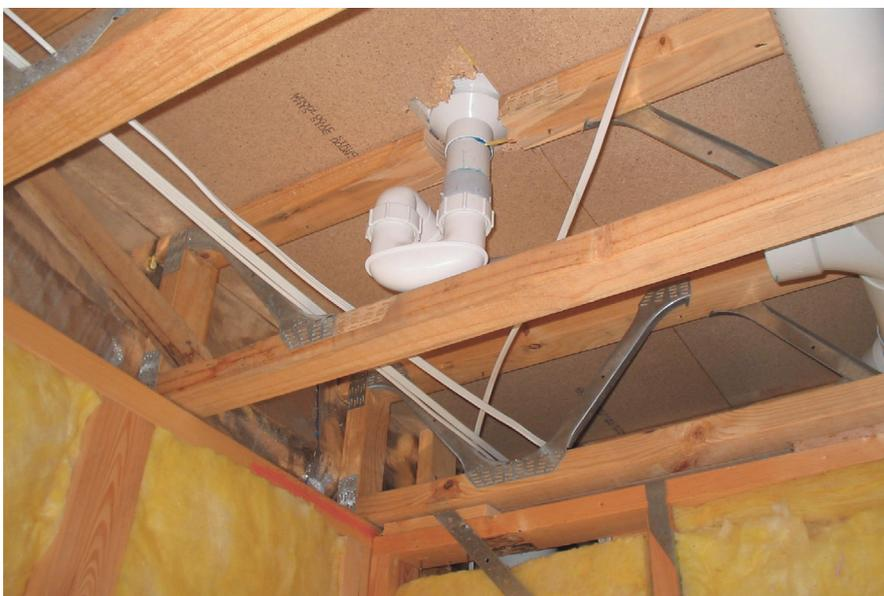
■ Floor truss cut and web removed to allow for services.
