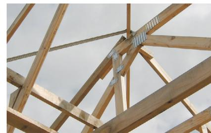
■ Section of truss has been removed and replaced with strap nails.
