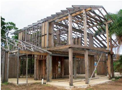
builder commonly neglects to have the trusses and wall frames checked by the truss manufacturer or engineer.
