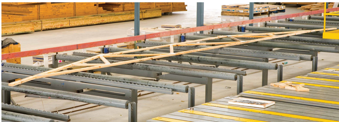
■ Many plants lack the space for truss outfeed rollers for safe truss removal.
