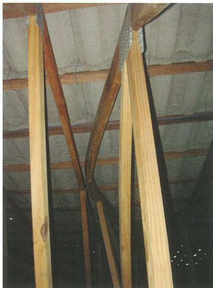
■ Girder truss failure - top chord restraints not fixed when girder initially installed.
