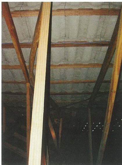
■ Girder truss failure - top chord restraints not fixed when girder initially installed.
