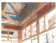
■ Typical connection to bracing wall.
