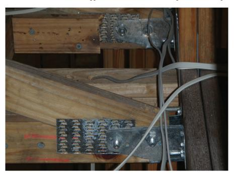
If trusses are supported by an internal wall, it is very important for every wall to be of the same height.
