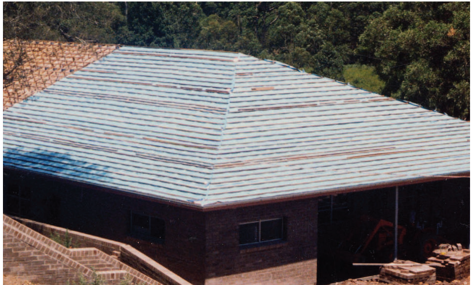
■ Sarking on the roof of a house.
