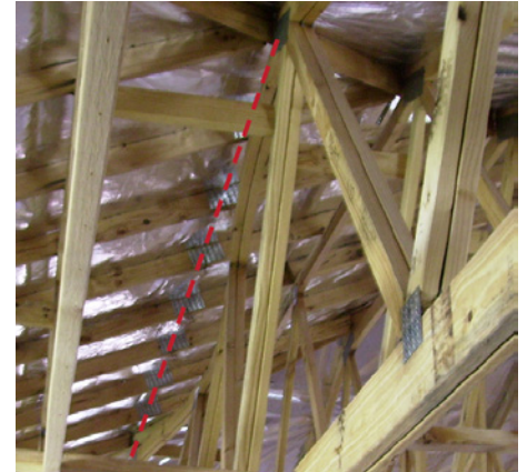
Photos 2 and 3: The buckled truss and truncated girder.
