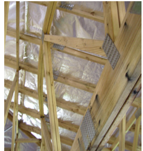
Photos 2 and 3: The buckled truss and truncated girder.
