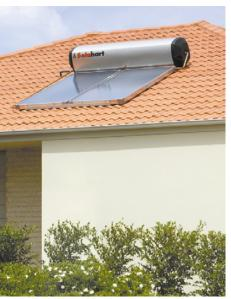
■ Typical installation of a SHWS and tank.
