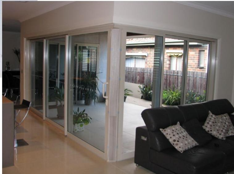
■ Photo 2: A corner post to support the header was missing.
