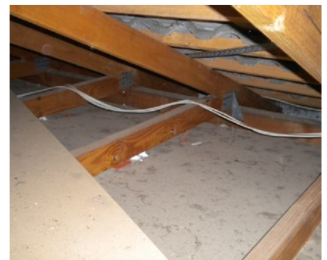
■ Roof space above roller door.
