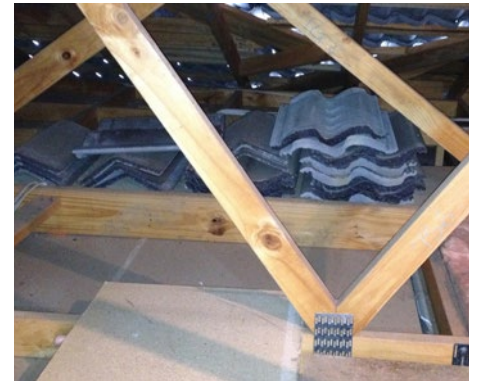
■ Surplus tiles stored in roof.
