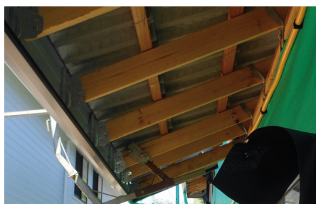
■ Typical guardrail post fixing to truss overhang
