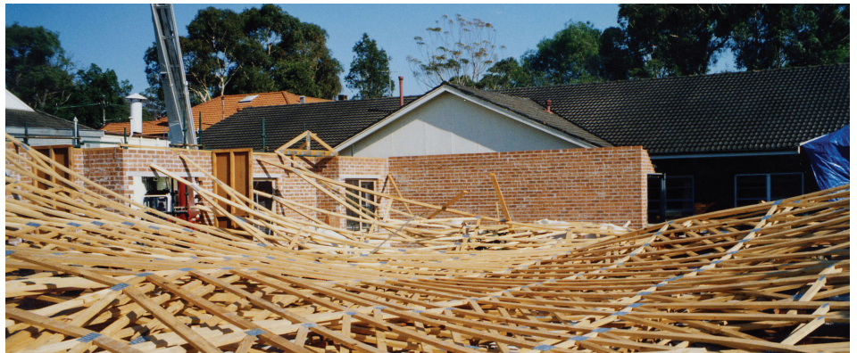
An example of collapsed trusses.
