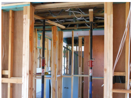
Image 2: The danger area was not closed off with any signs or barriers.
