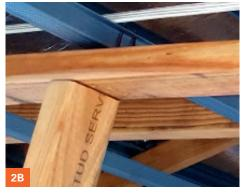
the battens will rest and bend over the wall causing ceiling and cornice cracking issues.
