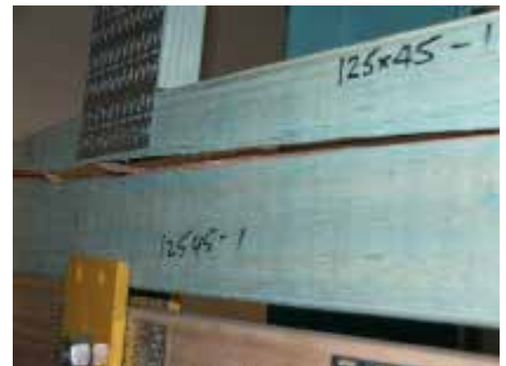
Figure 2: Tension perpendicular failure
