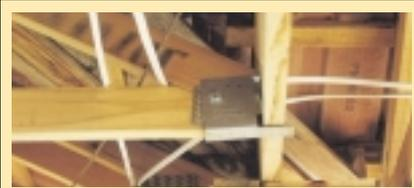
An exaggerated example of a twisted bottom chord due to incorrect bolting of the supported truss..
