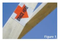
However if we have a series of trusses with the same fault, as we would have if a web brace was not properly installed, the chance of collapse is increased significantly.
