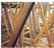
■ Web stiffeners should be used in preference to web ties where the webs to be braced are not in alignment.
