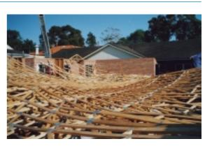
or "Speeedbrace" as temporary brace, which works well as a tension brace but has no compressive capacity so is the opposite problem to the nogging system.
