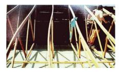
The correct installation and fixing of temporary bracing will help avoid these failures and provide a straighter and safer roof structure.
