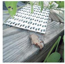
Prolonged exposure to weather causing timber splitting and joint failure.
