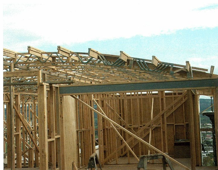
■ The curved roof in position, MiTek's Posi-RAFTERS completed the job design by architect Steve Hofer, utilising timber over steel in this instance.
