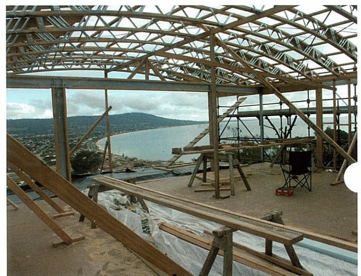
■ The curved roof in position, MiTek's Posi-RAFTERS completed the job design by architect Steve Hofer, utilising timber over steel in this instance.
